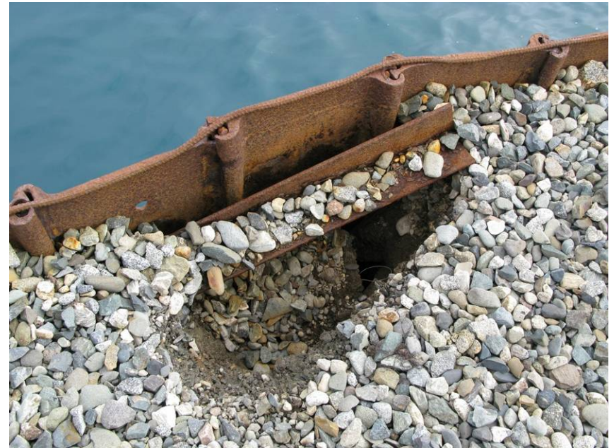
New Sink Hole 11/4/2008
